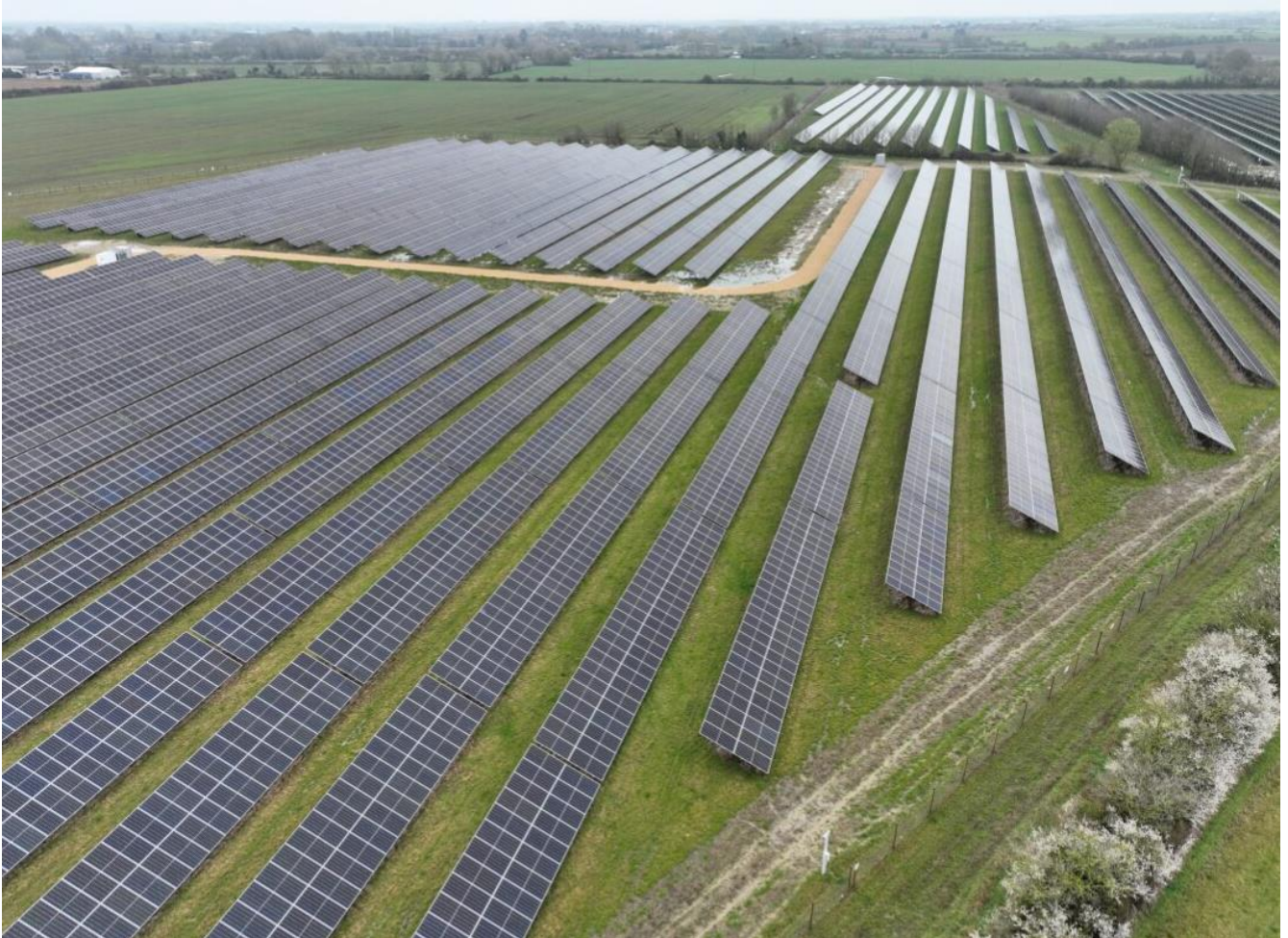
Plate 1: Typical Solar Panels
